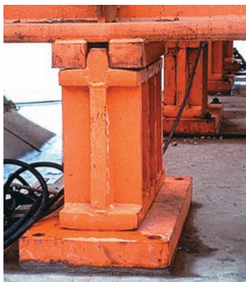
Photo 4.5 Shown is the rocker expansion bearing of a plate girder bridge. The convex surface of the rocker allows the support of the girder to move horizontally.
