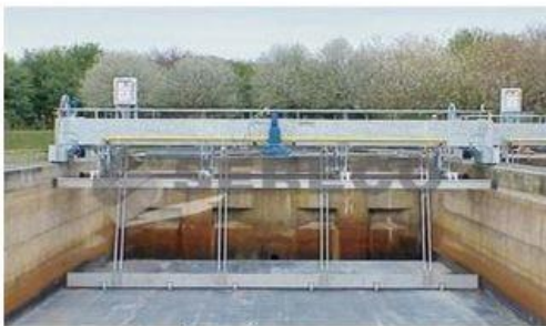
Bridge drive scraper
